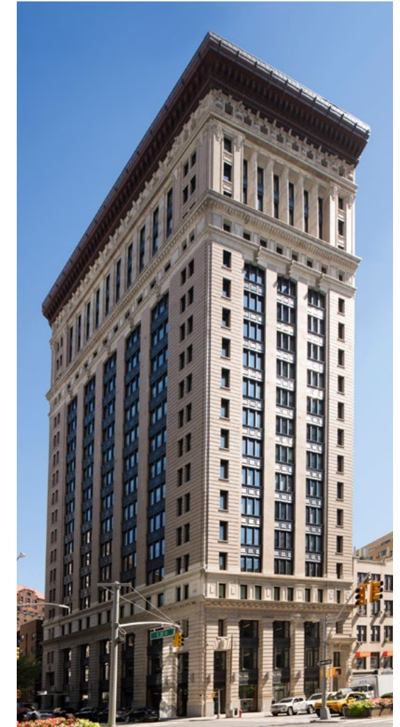
315 PARK AVE SOUTH
